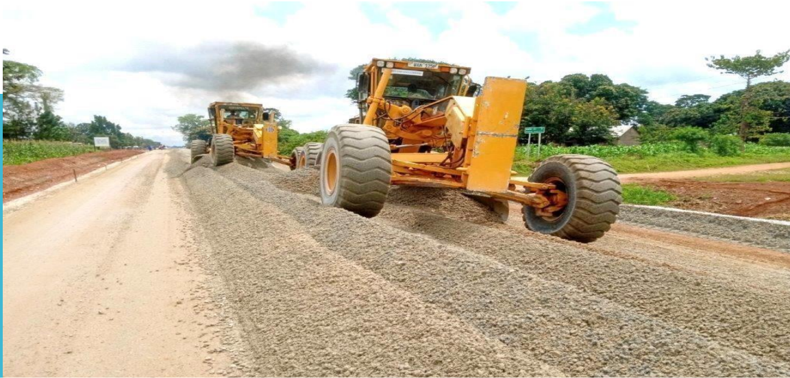
COMPREHENSIVE CRUSHED STONE BASE PREPARATION
