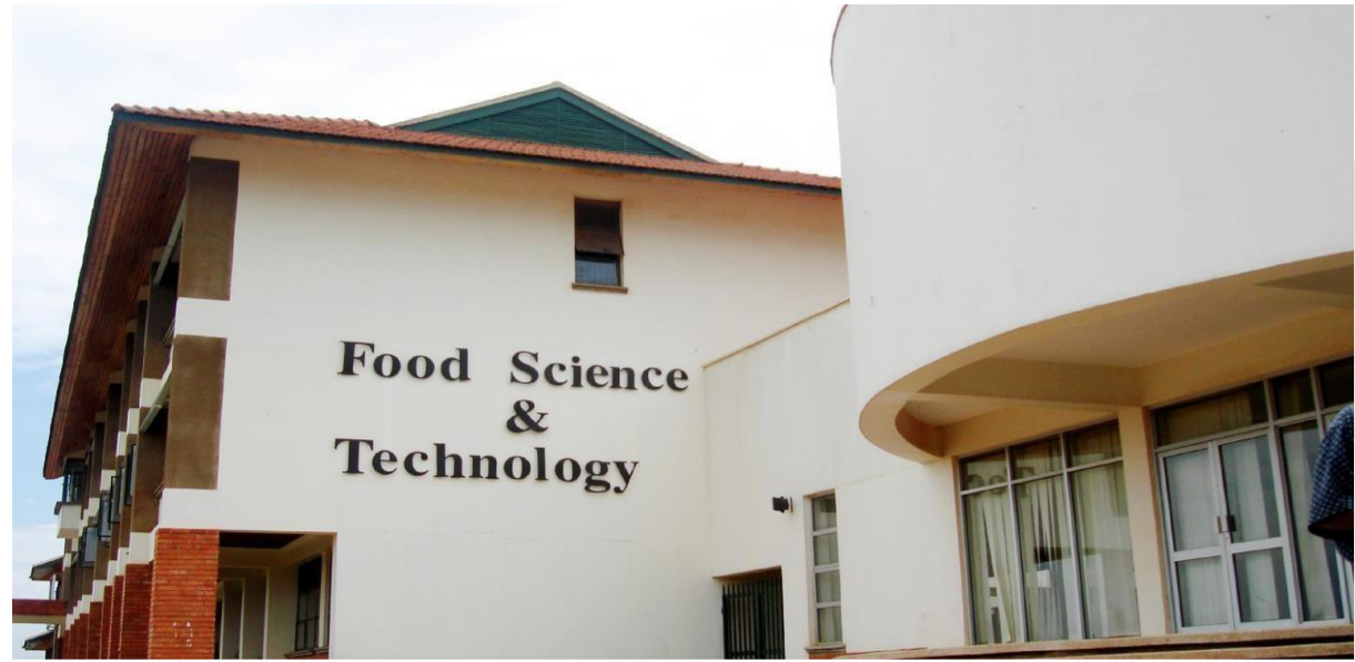
COMPLETED FOOD SCIENCE & TECHNOLOGY BUILDING COMPLEX - MAKERERE UNIVERSITY, KAMPALA CITY, UGANDA
