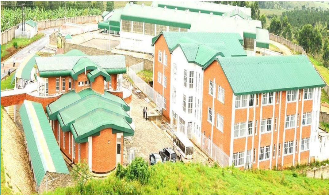
COMPLETED PIBID FACTORY BUILDINGS— BUSHEYNI, UGANDA
