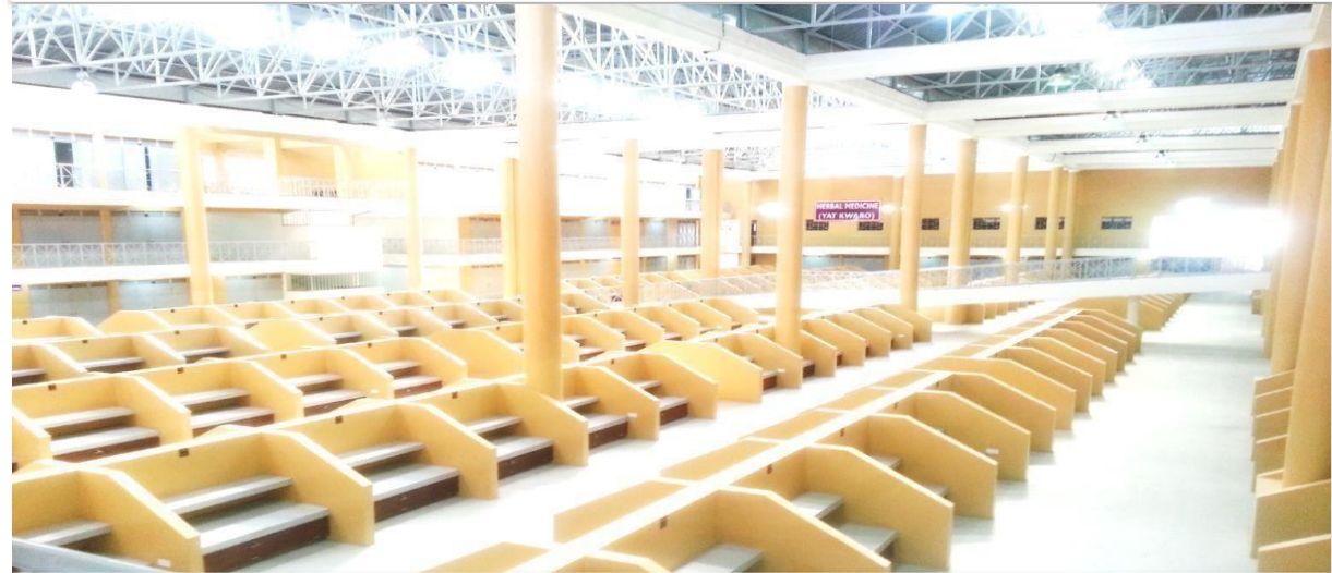
COMPLETED INTERIOR GULU MAIN MARKET COMPLEX, UGANDA
