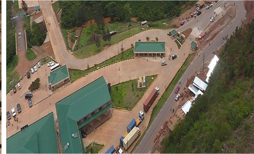
Constructed Mirama Hills Border Post
