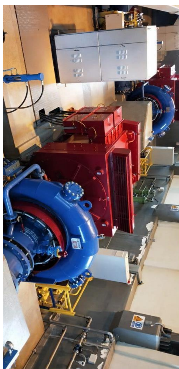
COMPLETED INSTALLATION OF TURBINES IN THE POWERHOUSE – WAKI, HOIMA, UGANDA
