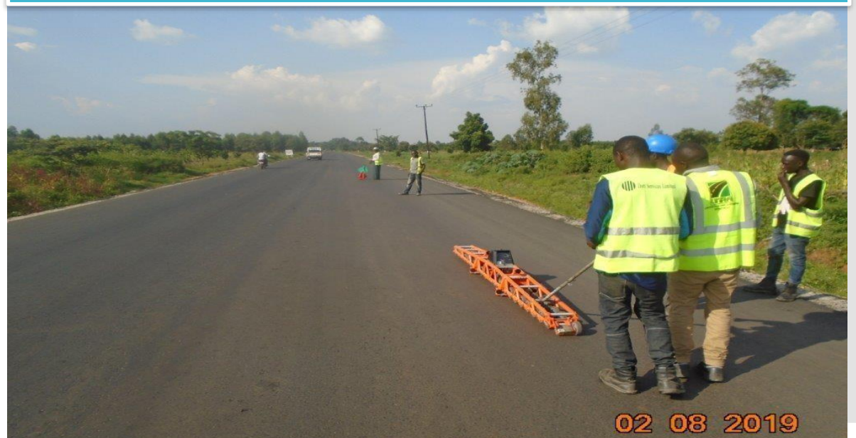
ASPHALT CONCRETE SURFACE RIDABILITY - QUALITY ASSURANCE/CONTROL
