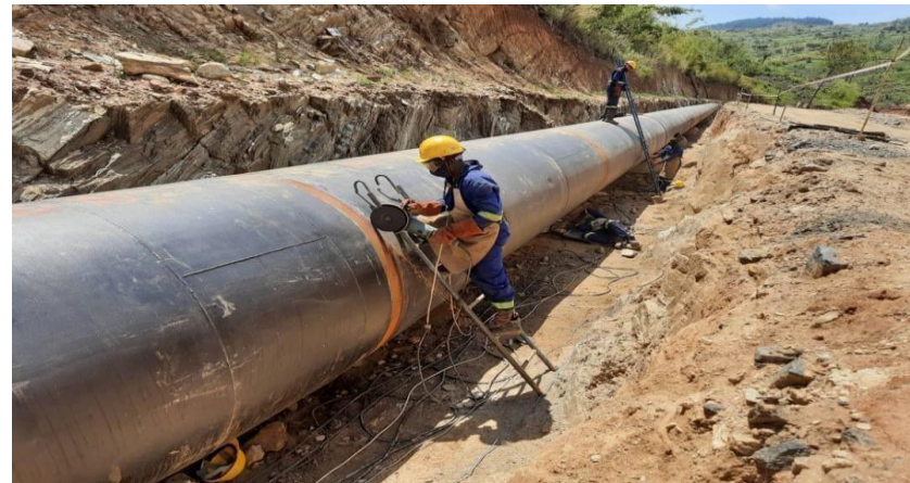
Steel pipe bending, rolling and installation
