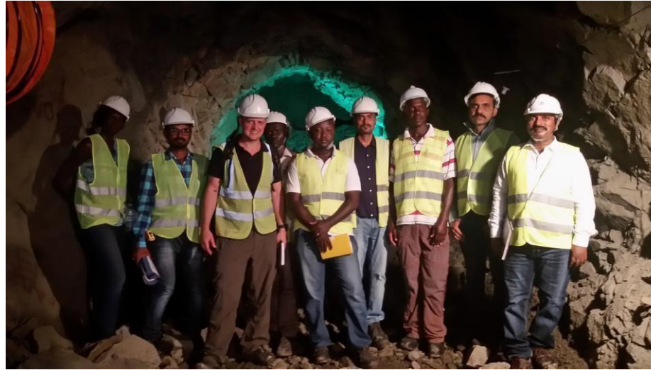
Tunneling at 4.8MW Waki Mini Hydro Power Plant
